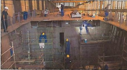
Project Funded: South African Shipyards – Ship building and repairs
